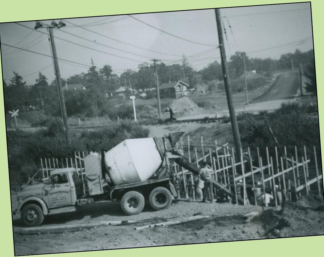
McKenzie Avenue Construction, 1968 (1980-015-038i)
