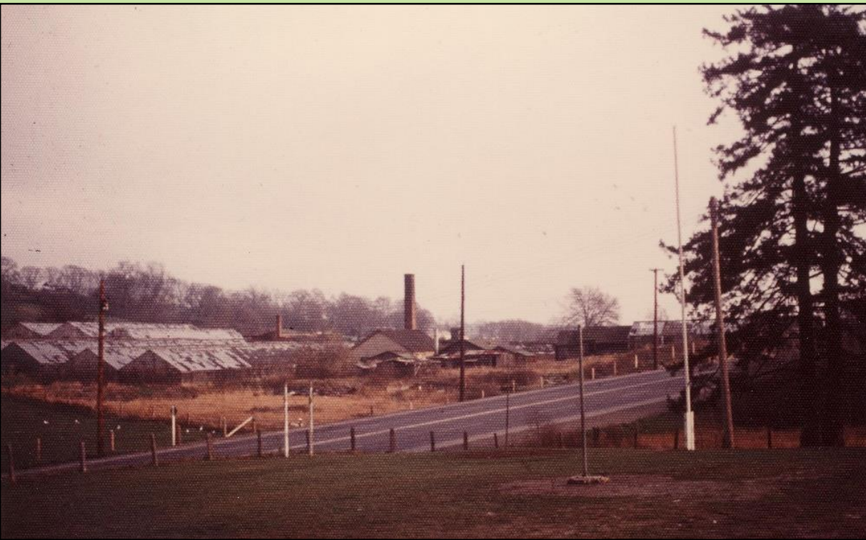
Lum greenhouses, Douglas Street, ca. 1960s (1978-001-072)
